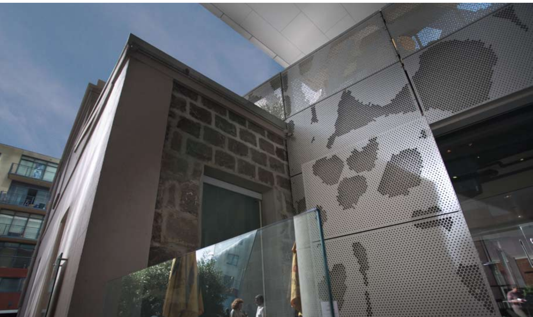
The main building blends well with the old and new. The outdoor living area is designed to make the most of this interesting context.
